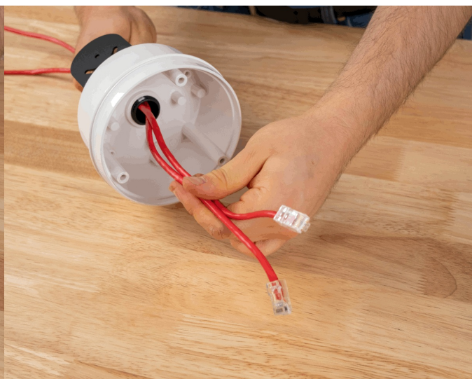
View of cable for service loop
